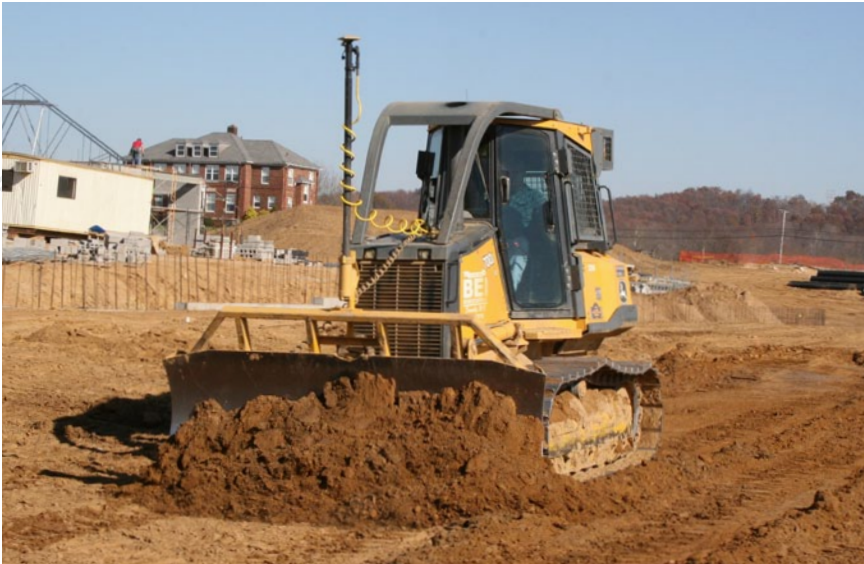
Brown estimates that Topcon's 3D-MC2 system will probably knock four to six weeks off the project length, largely because of gains they've made in final grading.
